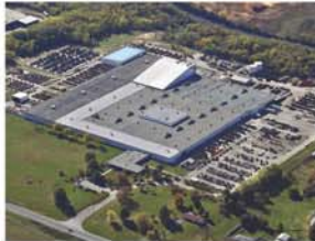
Richmond, KY - Manufacturing Plant
