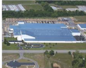
Orangeburg, SC - Manufacturing Plant
